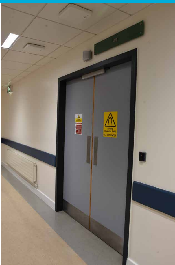
Patient movements are captured by means of RFID readers installed at doorways.
